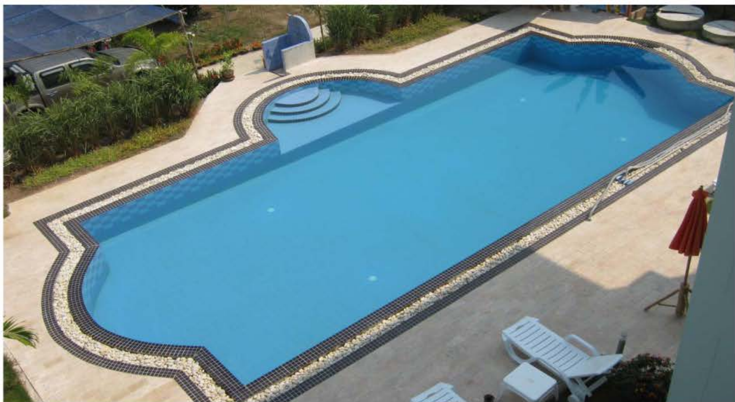
Pool with roman steps and overflow channel, about 15.0 x 7.5 m.
