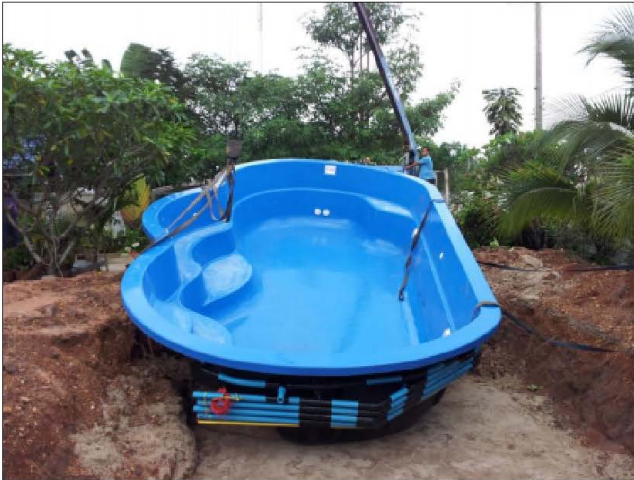
Setting the pool into the hole
