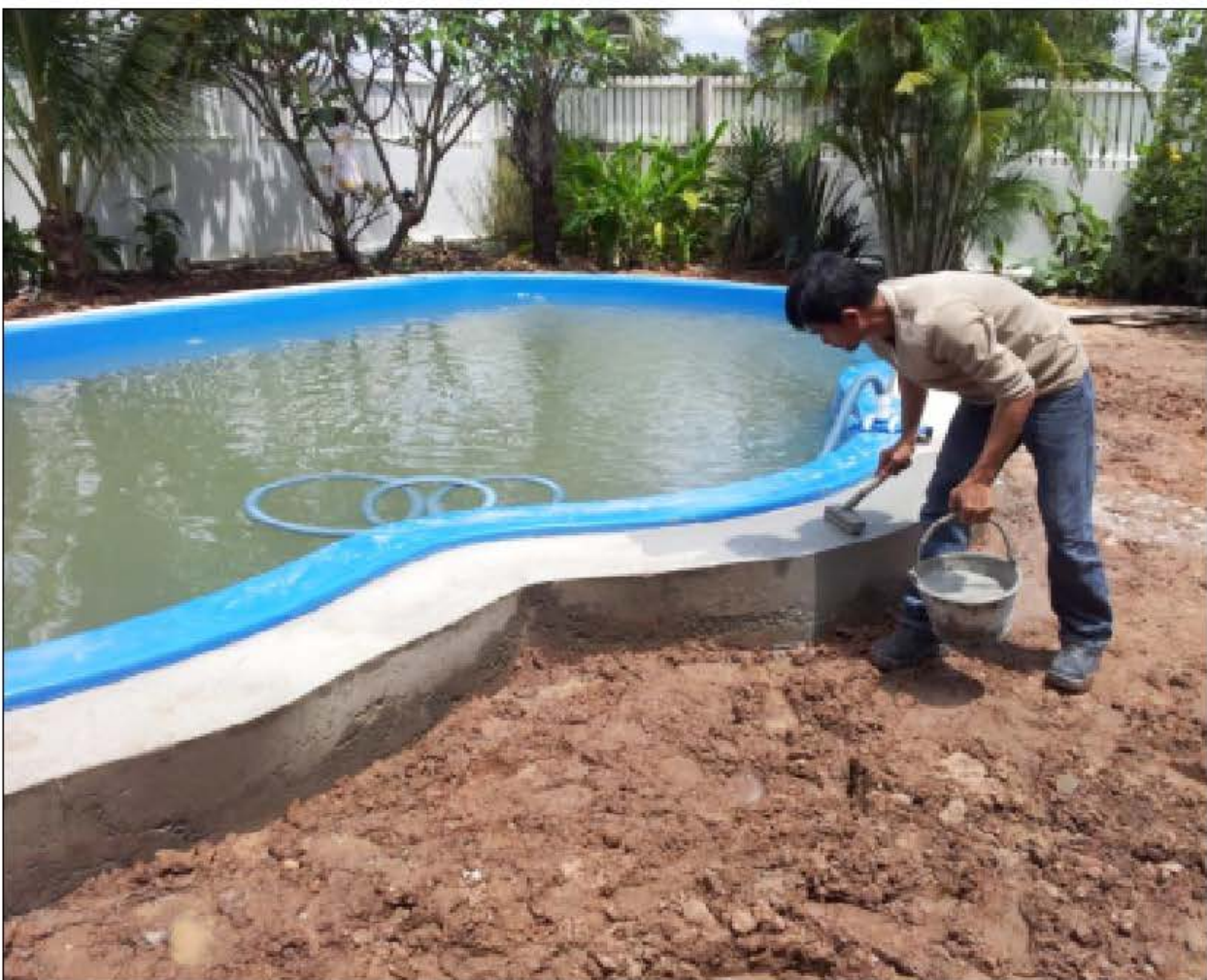
Pouring the concrete for the surroundings
