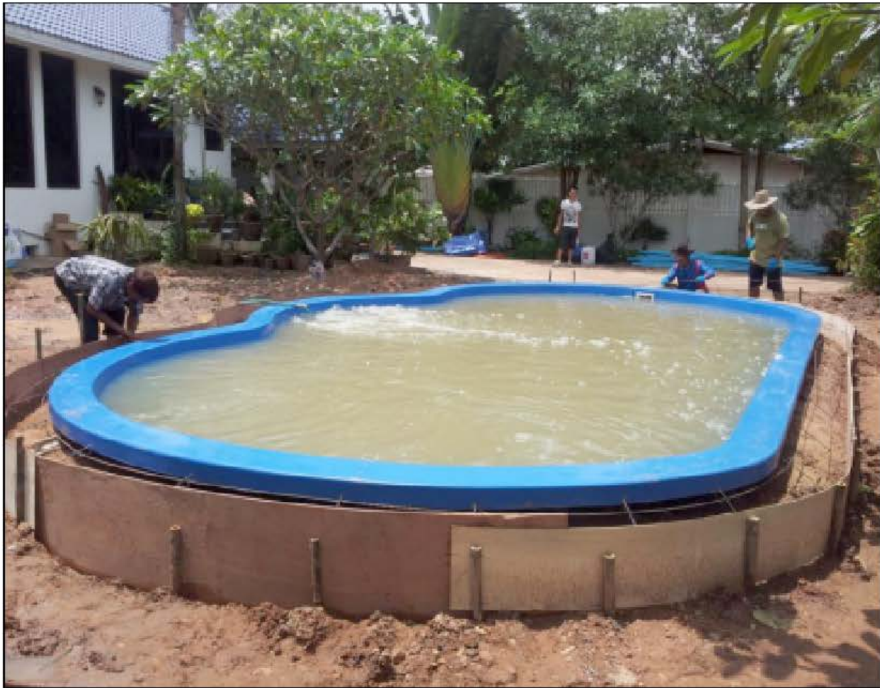
Filling the pool with water and preparing the casing
